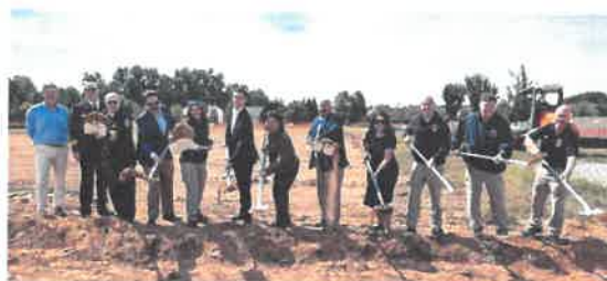
Wake County and Town of Fuquay-Varina recent ground breaking of new fire/EMS station.
