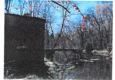
Existing Pump Station
