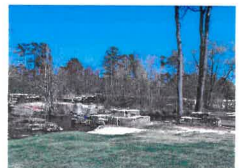
Moore's Mill Building Foundation along River
