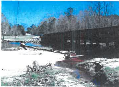
Daylighted Stormwater Channel
