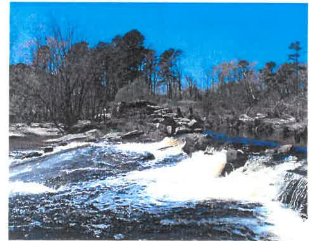
Existing Condition of Moore's Mill Dam
