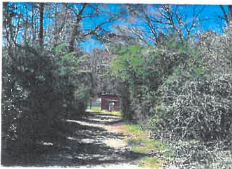
Path Leading to Pump Station
