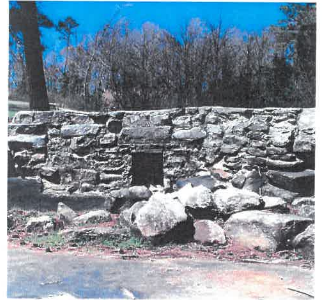
Western Portion of the Dam
