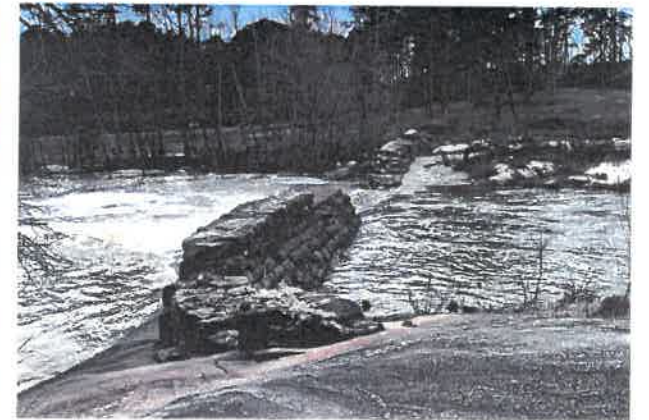
Dam Structure from the Eastern Side of the Park
