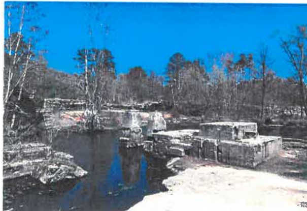
Support Structure Foundations and the Mill Wheel Holders
