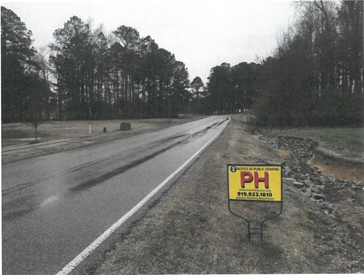
Posted Sign Looking South on Industrial Drive
