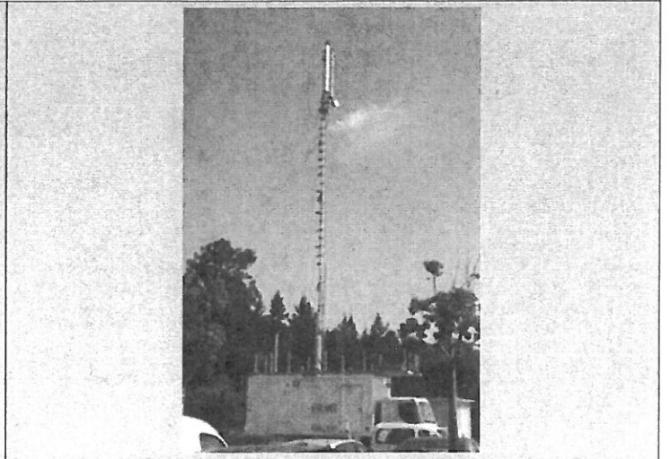
Temporary facility in a vehicle
