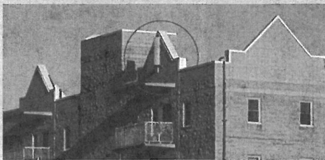
Concealed collocation on a building (red circle added for clarity)
