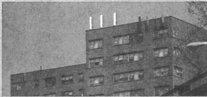
Typical collocation on a building
