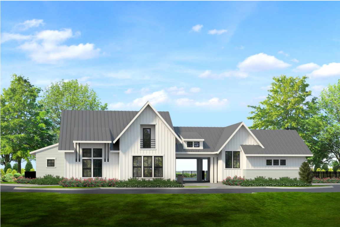
Site Amenity (Front View)
