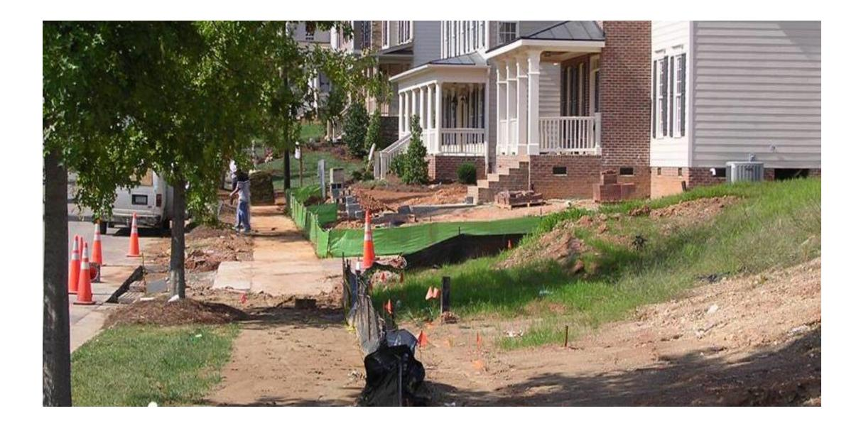
What is it? Silt Fence not working properly allowing sediment loss.
